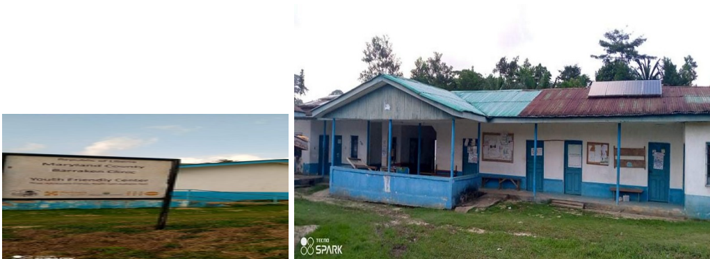
Figure 12: Barraken Clinic, Barraken Town, Maryland County.
